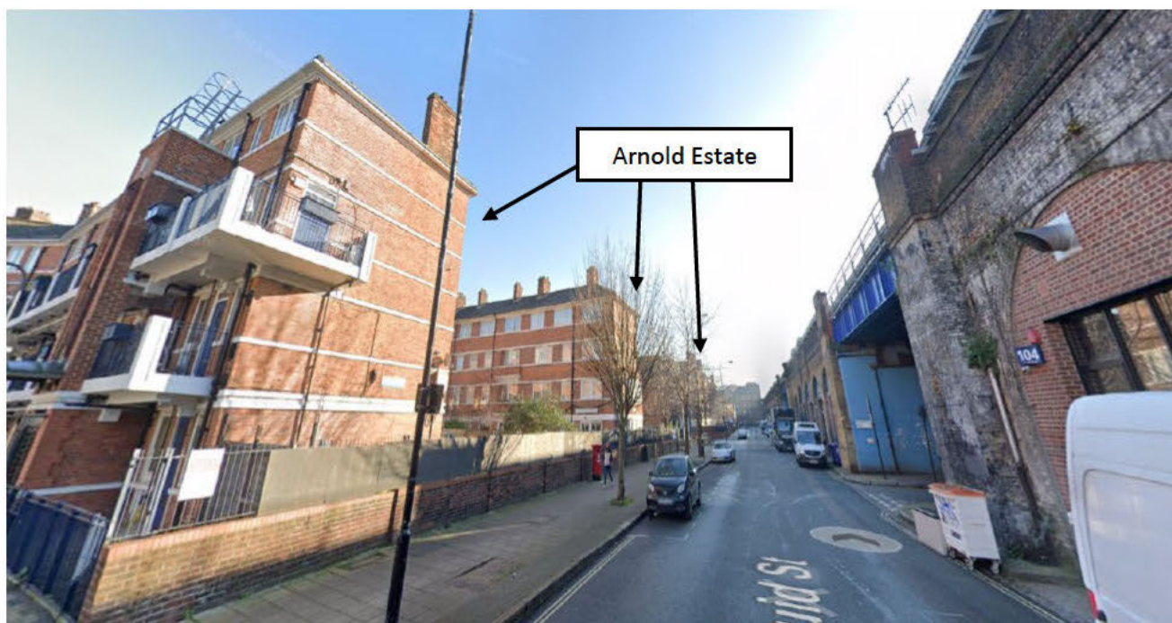
Figure 4: View looking south west down Druid Street showing the Arnold Estate
